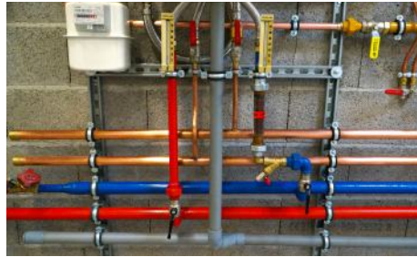
PLUMBING & SANITARY WORKS
